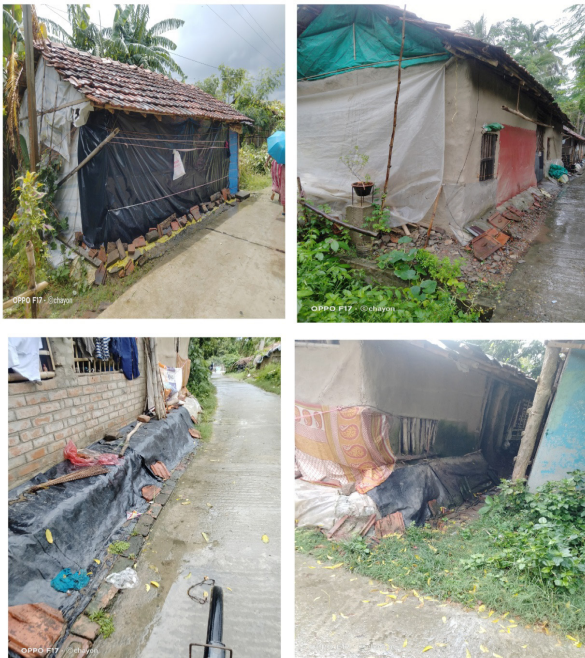
Fig 12: Protective measures for kuccha houses
